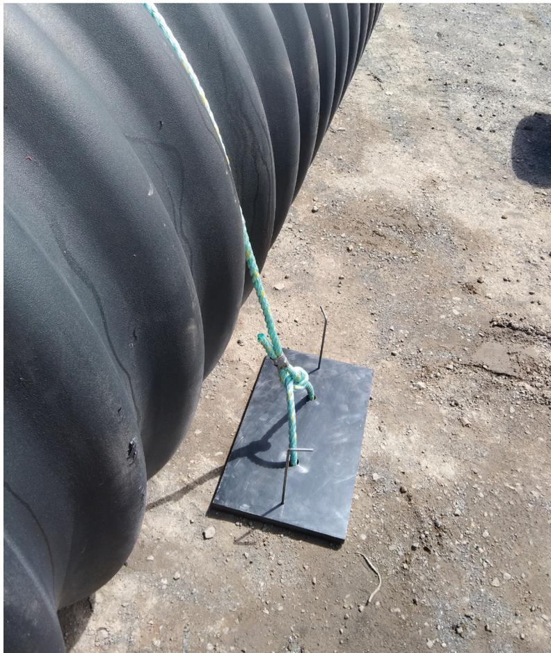
This is an indicative photo to show the placement of the pads and the tightness of the rope. It is not an actual install as there is no trench or compacted basecourse shown.
