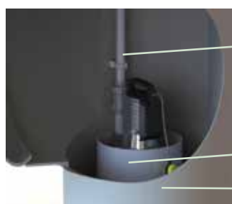
Submersible Pump Option + Tank Internal Pipework & Pump Platform
